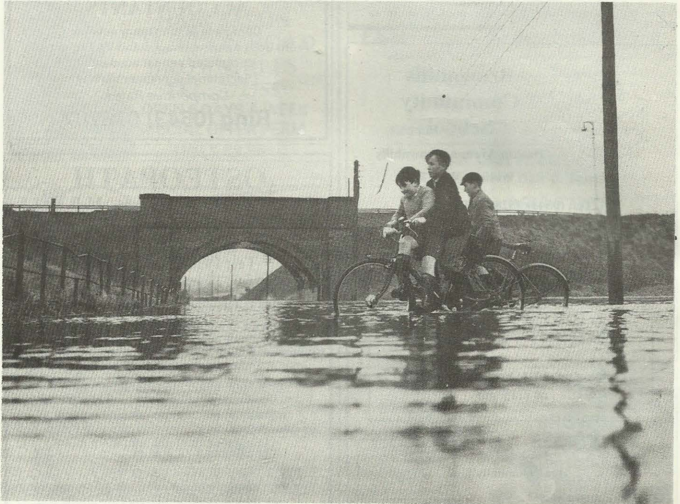
CLAYHANGER RAILWAY BRIDGE FLOOD
